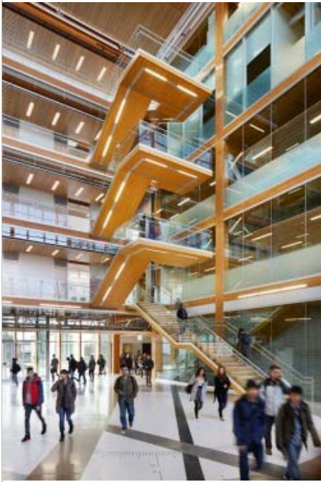
The north wing of the University of British Columbia' Earth Sciences Building (ESB) uses glulams in its columns and beams, laminated-strand lumber in its floor panels, and cross-laminated timber for its roof and canopies.
