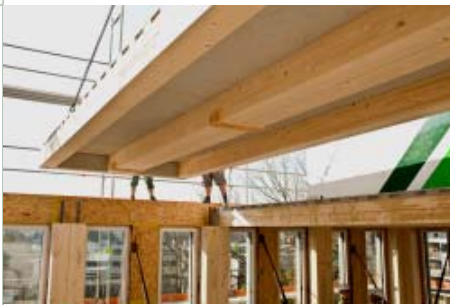
CREE's LCT ONE uses a hybrid system that incorporates glulams and concrete into the floor and wood walls that are pre-assembled in their factory and then assembled onsite.
